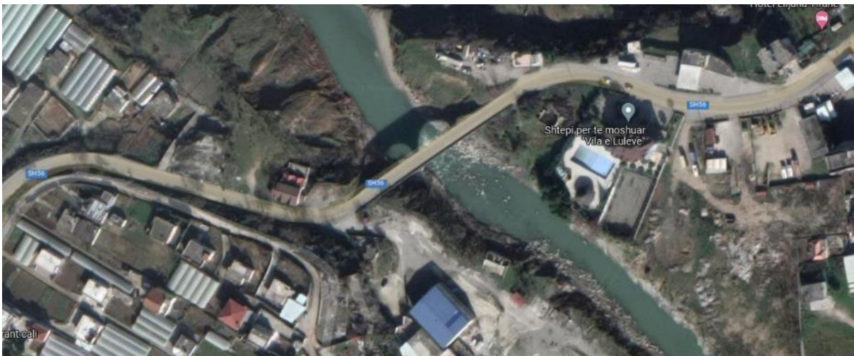
Bridge over the Erzeni River – top view
