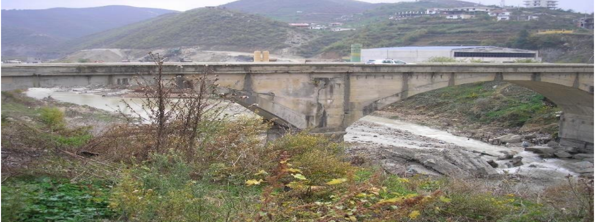
Beshiri Bridge over the Erzeni River – side view
